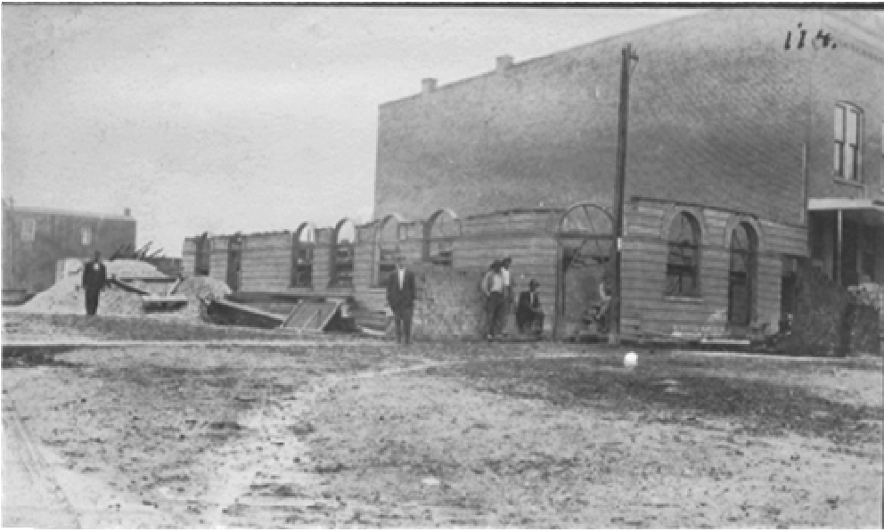
Northeast corner of Main and Palmyra streets under construction for the new Peoples bank
