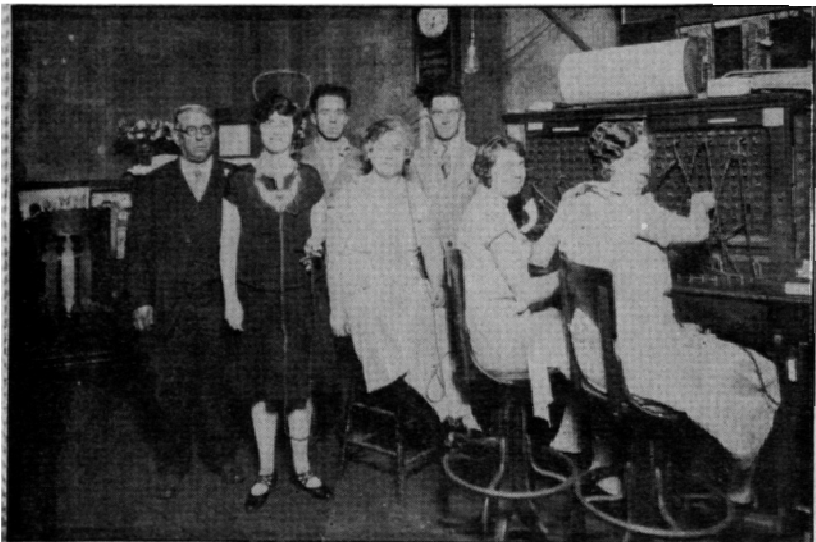
CALL WAITING: Telephone service came to Perry around 1901. This turn-of-the-century photo shows the Perry switchboard and the people who operated it. The young man in the middle was Nelson Stehle, who had a part in the Perry exchange until 1928. At the time this photo was taken, the switchboard was operated from Stehle's home.
